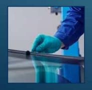
Before use, shake the **DINITROL 538** Plus one-step primer (bottle) for approx. 1 minute until the steel ball is audible. The aluminium tube does not contain a steel ball, but the tube must also be shaken well before use. Now use a dauber or the tube to evenly apply one layer of primer to the clean bonding surface.
