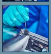
Paint damage on the flange can be touched up with **DINITROL 538** Plus one-step primer. Before touching up, shake the bottle for approx. 1 minute until the steel ball is audible or shake the primer tube (without steel ball) for approx. 1 minute as well (see Figure 5).
